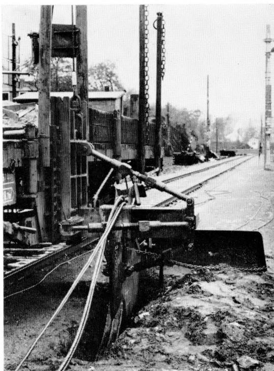
Figure 12—Plowing the cable into the ballast of the railway line.
