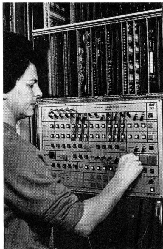
Figure 5—Control panel of the central processor.
