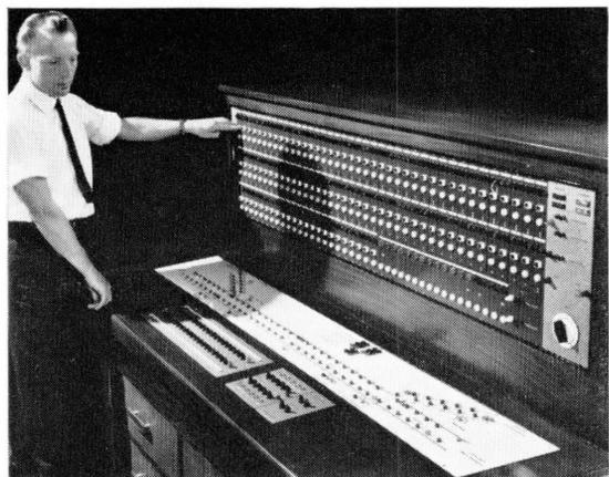
Figure 12—Console for the alarm system to report fires and accidents in the Mersey tunnel.
