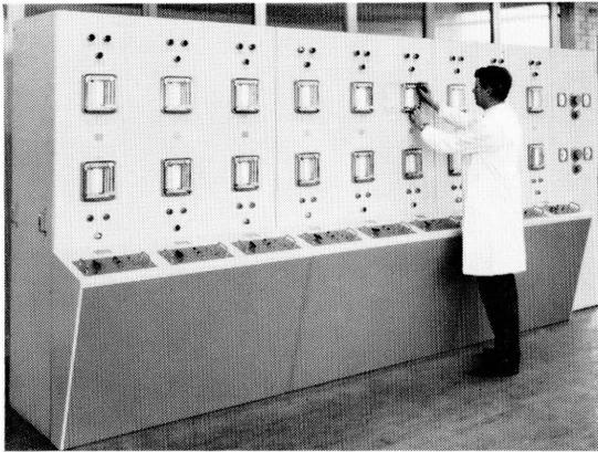
Figure 3—Control-room instrument panel with controlling recorder stations and alarm system.
