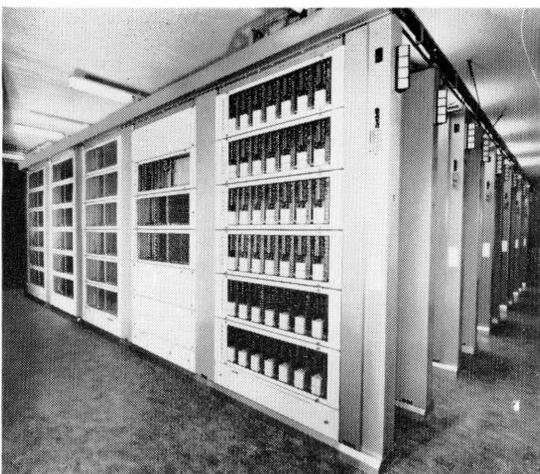
Figure 11—Regensdorf Pentaconta exchange in Switzerland.
