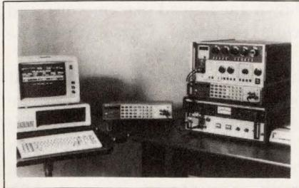
also checks dc-voltage, ac- and dc-current, and resistance functions. The system uses the company's 1605A transfer standard and an IBM PC fitted with an IEEE-488 board to control the calibration system. The system software works with a variety of calibrators. From \$29,000. Delivery, four to eight weeks ARO.
