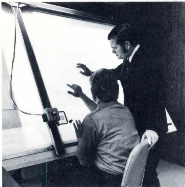
Fig. 5—Digitizing a chip cell plot at Motorola's Localogic center feeds cell location, metallization and chip-pad locations to key punch. Control cards are then used for generating fabrication masks.
