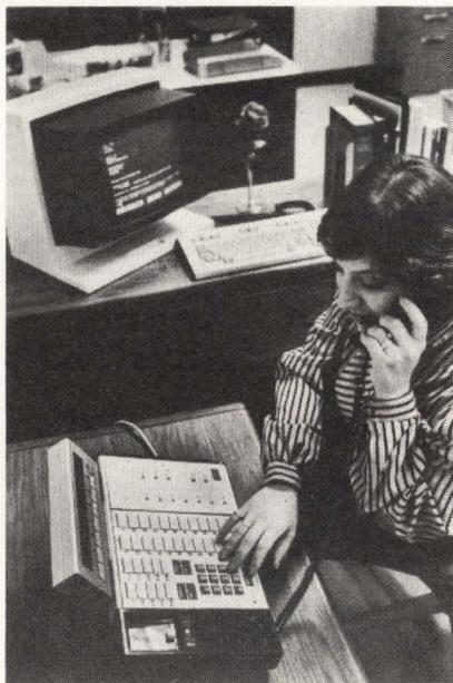
The System 75 communications system combines voice, high-speed data, and communications and system management features into an integrated system. It is designed for installations of 300 lines and can be upgraded. The system 75 can transmit voice and data simultaneously over one line at 64,000 bps. The system has a system management capability for customization in different applications such as diagnostics. **AT&T**, Morristown, NJ **Write 130**
