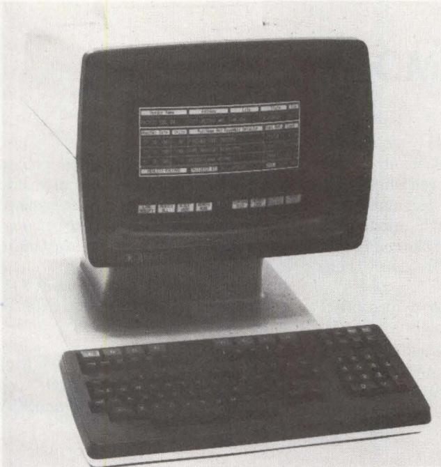
modify and character modes, with full-duplex async data communications. Computer connections are via RS-232-C interface, with an optional 20mA current loop. The HP 2622A display terminal is \$2,075. Integral thermal printer is \$1,210, the line-drawing character set is \$105. **Hewlett-Packard Co** 1507 Page Mill Rd., Palo Alto, CA 94304. **Circle 203**
