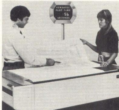
ings in less than 30 seconds. An 11-inch model can plot directly from a display terminal and can also perform computer-directed work. Unit produces scientific graphs, business PERT charts, maps, production drawings, engineering simulations, and circuit designs. Shadings, tone patterns, and varied line widths can be combined with printing of captions, legends, and other alphanumeric data. Versatec, 2805 Bowers Ave., Santa Clara, CA 95051. (408) 988-2800. **Circle 209**
