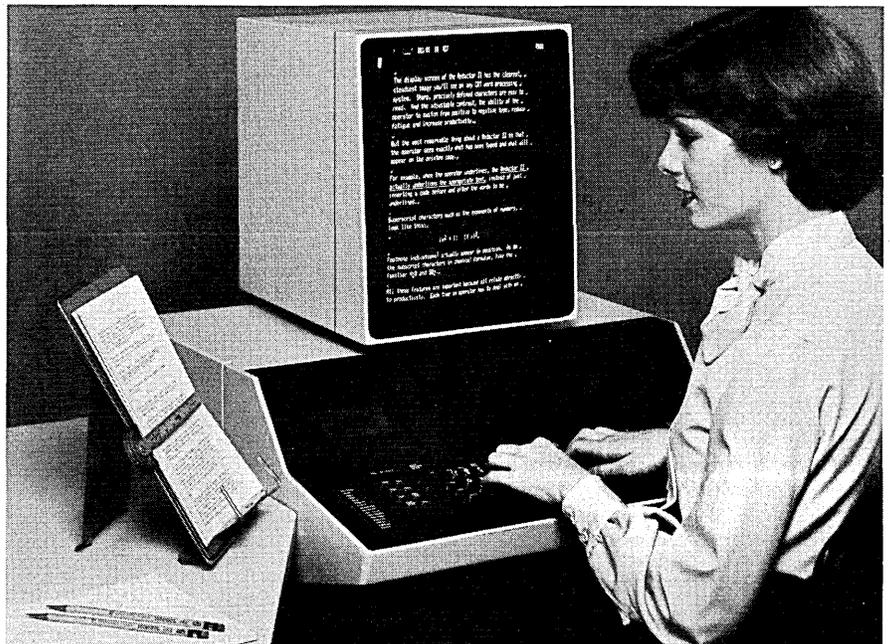
Where word processing systems differ rather strongly from data processing systems is in the need to display the text being produced exactly as it will appear in print. This requirement leads to large displays capable of handling functions like superscripts, subscripts, and underlining, as this unit from Burroughs/Redactron is here.
