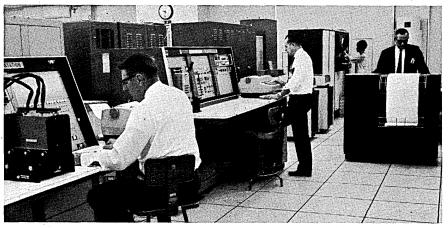
controlled system of automatic checkout equipment shown in the accompanying diagram and photographs. The system provides an improved test and fault isolation capability for the analog and digital assemblies which comprise the avionics systems manufactured at their Woodland Hills, Calif., plant.
