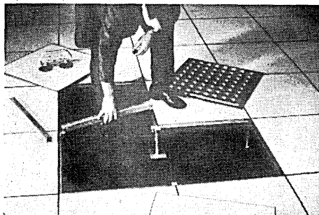
Stringers are easily removed from the exclusive Snap-Lok Rigid Grid System.
