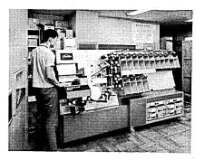
fonts as ISO-A and -B, IBM, NCR, Farrington 12 F and the Toshiba Stylized Font. Characters are recognized by their geometric features rather than stroke, thickness, or position. Main components are a paperfeeding mechanism, photoelectric scanning device, and i.c. recognition logic. Width of the journal tapes can range from 56 to 100 mm.
