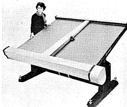
a speed of over 700 inches/minute. The system has an accuracy of  $\pm 0.002$ -inch and resolution of .001-inch. DDS has computerized logic, a non-destruct memory and modular design.
