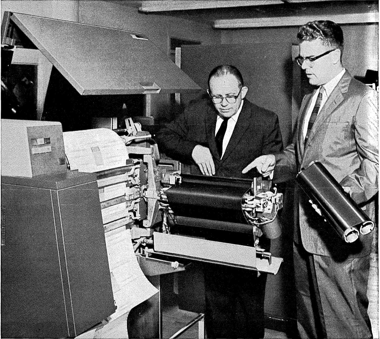
Messrs. Faulkner (left) and Jones examine Columbia SF-100 Mylar Ribbon in high speed chain printer at Spiegel, Inc. computing center.
