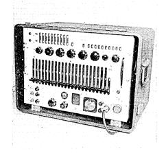
puts include precision time as a 28 bit binary number, a pulse which occurs at a preselected time and WWV audio signals. AC input power can be 60 or 400 cps, and an internal inverter allows power input from 24V DC source. GENERAL MILLS, INC., 1620 Central Ave., Minneapolis 13, Minn. For information:
