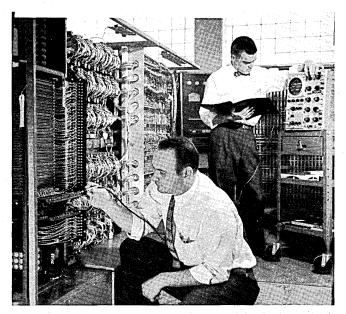
Bow holds a probe on one of the signal leads for a 705 core memory unit while Durkin checks the oscilloscope pattern against the reference pattern in the Central Processing Unit book.
