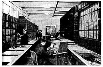
mathematic expression of the laws governing the passage of electric current through conducting plates. Thirty thousand different values representing the natural factors operating in the deposit can be introduced into the machine.
