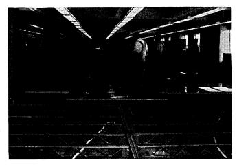
N. Y. Telephone Co., New York City employs approximately 18,000 square feet of Macomber Computer Platforms to support IBM billing machines in its New York Coliseum Building Accounting Department. Problem was to distribute and transmit uneven weight load to building steel. Although load averaged 25 lbs. per square foot, concentration of machines in some areas, boosted load to 200 lbs. per square foot. Macomber Computer Platforms solved this floor load problem.
