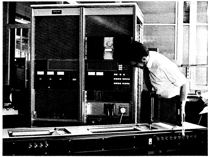
Figure 3 - TXE4 switching exchange printed boards being checked out using PROTEST language to control the test routines at STC's factory, New Southgate, England. The PROTEST tape can be seen in the top right hand corner of the tester. The compiler and software are situated at ITT Data Services and can be reached by the test personnel using normal telephone lines.
