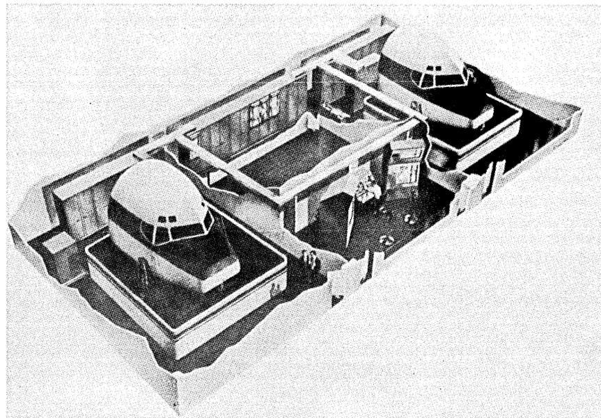
— The two replicas of the Boeing 707 flight deck will operate from the single digital computing source, the Link GP-4 and a three-million bit Bryant Computer Products Drum memory.
