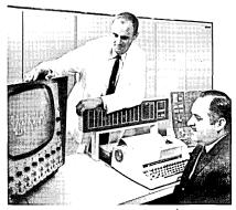
— Dr. Richard Yoder of Tulane University discusses the brain wave signals displayed on a cathode ray tube monitor with W.J. Nettleton, Jr., assistant director of the Tulane Bio-Medical Computing System Center. Mr. Nettleton is seated at the console of an IBM 1410 which is being used to analyze electroencephalogram wave forms.
