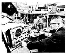
A fully operative model has been built but not fully complete (shown in above photo). It has a full read/write cycle time of 240 nanoseconds and a bit-rate frequency of 114 mc.
