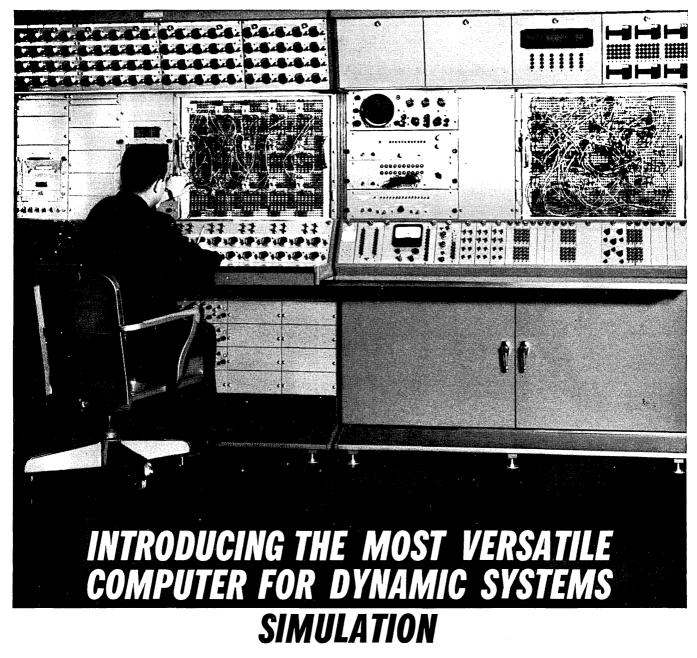
EAI HYDAC Computer, Series 2000, introduces a new dimension to computer simulation by combining analog and digital operation into one integrated system. HYDAC achieves a computational efficiency well beyond the limits of either analog or digital computers alone. Moreover, it offers an economical alternative to tying a complete data processing computer to an analog computer for hybrid computation.
