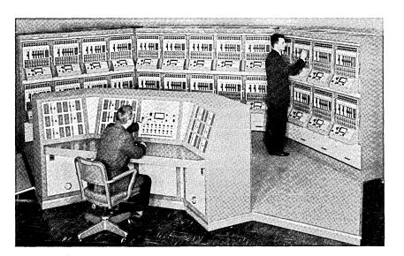
ANALOG COMPUTER SYSTEM FOR U.S. SIGNAL CORPS Electronic Associates, Inc. Long Branch, N.J.
