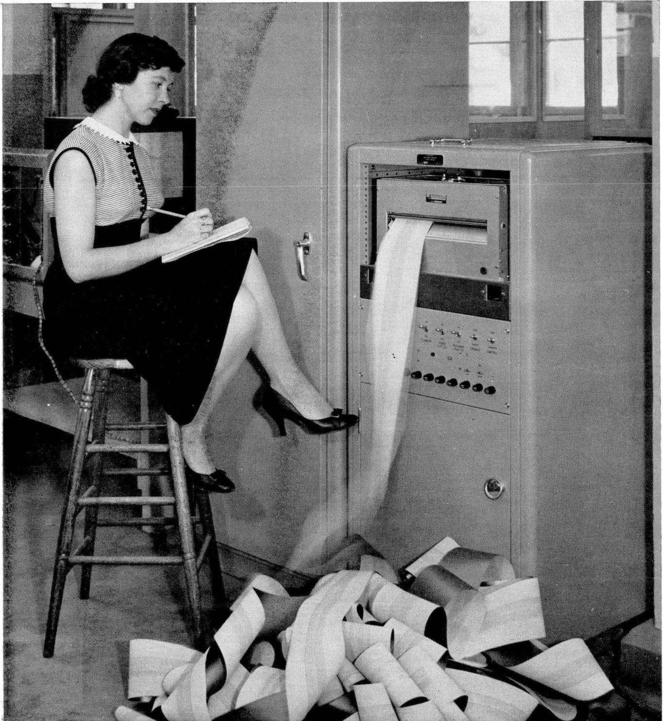
A digital printer, made by Radiation Inc., Melbourne, Fla., which produces 180 lines of printing per second, each line containing 12 numeric characters. The paper issuing from the machine is electrosensitive, marked by current passing through it. Each numeric digit consists of a selection out of an array of 30 points, 5 wide by 6 high. The speed of over 2000 characters per second is only about 500 times faster than a human being. (Figure 28)
