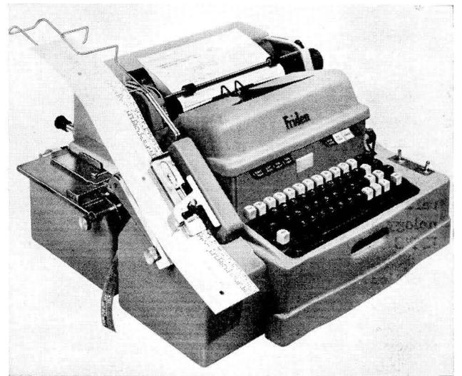
A machine which types a purchase order or other basic record, and at the same time punches paper tape or cards — a combined input-output machine. This is the Flexowriter, made by Friden Calculating Machine Co., San Leandro, Calif. (Figure 31)
