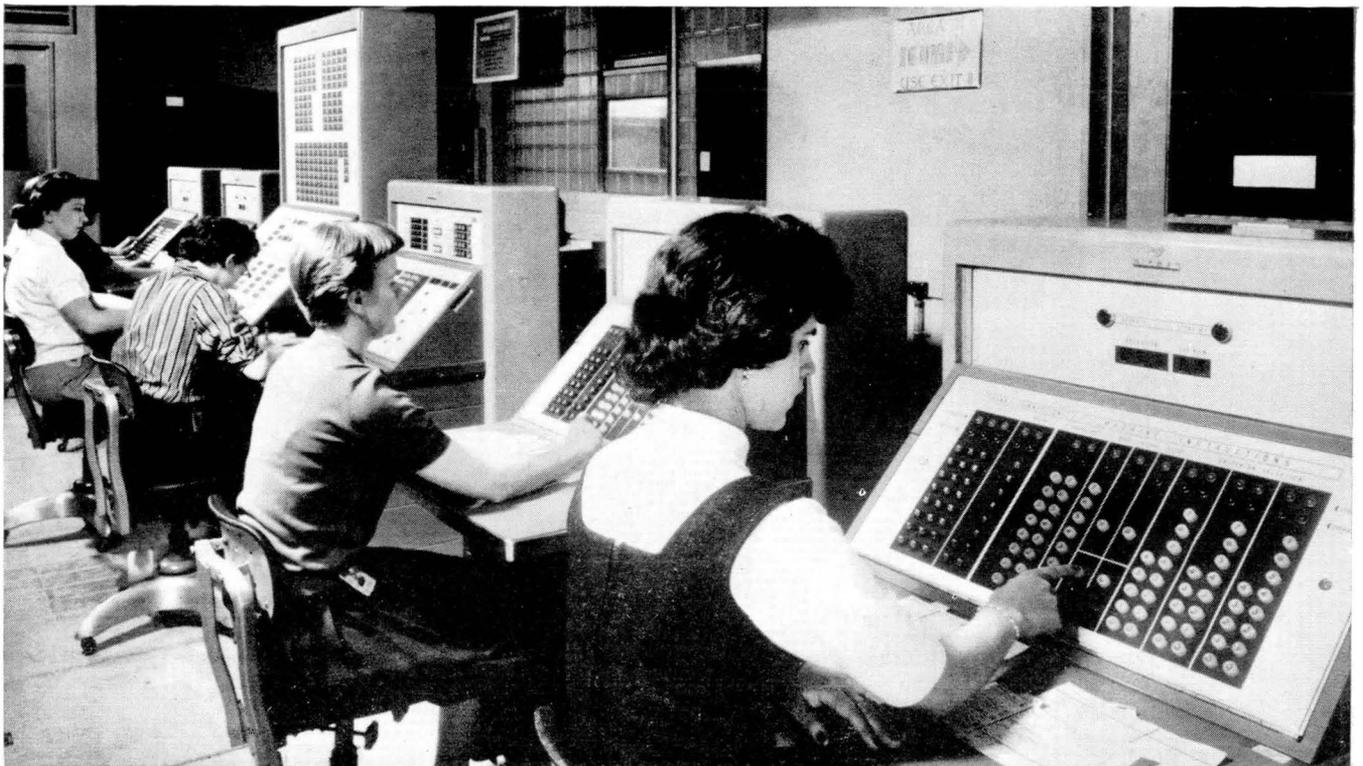
The "System Central" of the RCA Bizmac in Detroit, which functions like a telephone exchange. An operator at any one of these consoles can connect any of the 182 magnetic tape stations to the appropriate data processing machine by pressing a button; and she can tell from a glance at the control panel which machines are busy and which can take on a new job. (Figure 4)
