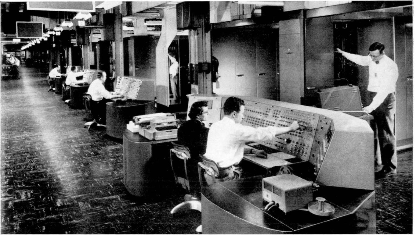
Operating the Bizmac, a very large automatic electronic computer, made by Radio Corporation of America, and installed at the Detroit headquarters of the Army Ordnance Tank-Automotive Command. The Bizmac system includes about 220 units of nineteen different types of equipment. (Figure 3)
