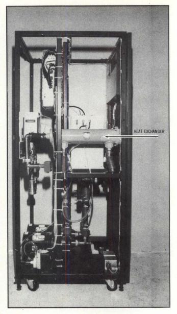
Photo 4 A remote heat exchanger unit contains pumps, bypass valves, and temperature and pressure monitoring circuitry.
