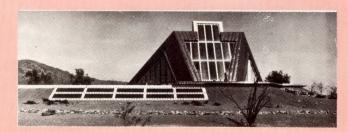
Fig 1 South elevation of Ahwatukee House. Solar collectors are used for heat and hot water, and earth berms piled against outside walls provide insulation. Windows have been eliminated wherever practicable, but special skylights permit use of sun for daytime lighting
