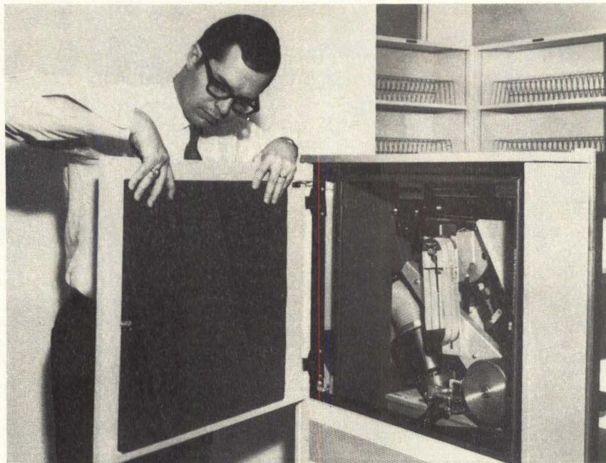
Rear-door view of RCA printer shows one-inch-thick SCOTTFELT on inside of door panel and on interior surfaces, where it forms a barrier to escape of noise from inside printer mechanism. The compressed polyurethane foam material, developed by the Foam Division of Scott Paper Co., is also used on air intake and exhaust sections of the printer to help achieve a 25-decibel reduction in the speech interference level
