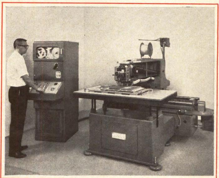
blocks, bus bars, cable connectors, junction blocks, relay blocks, and other devices. Furthermore, large-scale wiring of these products may be accomplished by mounting them on a panel and programming the TERMI-POINT machine for high-speed automatic wiring.
