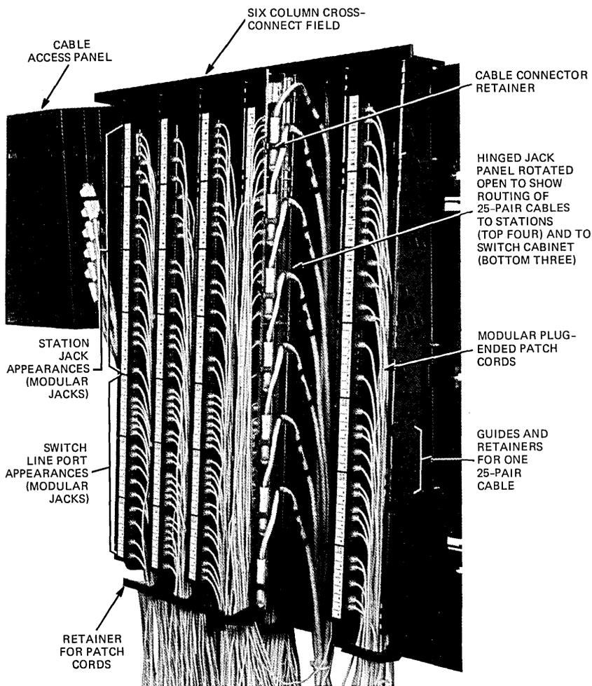
Fig. 11—Modular-jack-based cross-connect field.
