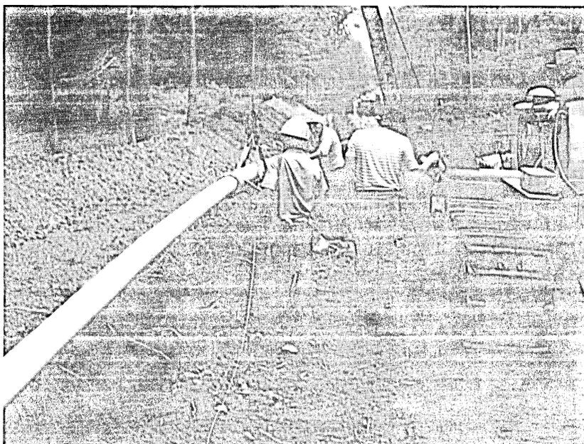
Fig. 8—Sheath being lowered into trench.
