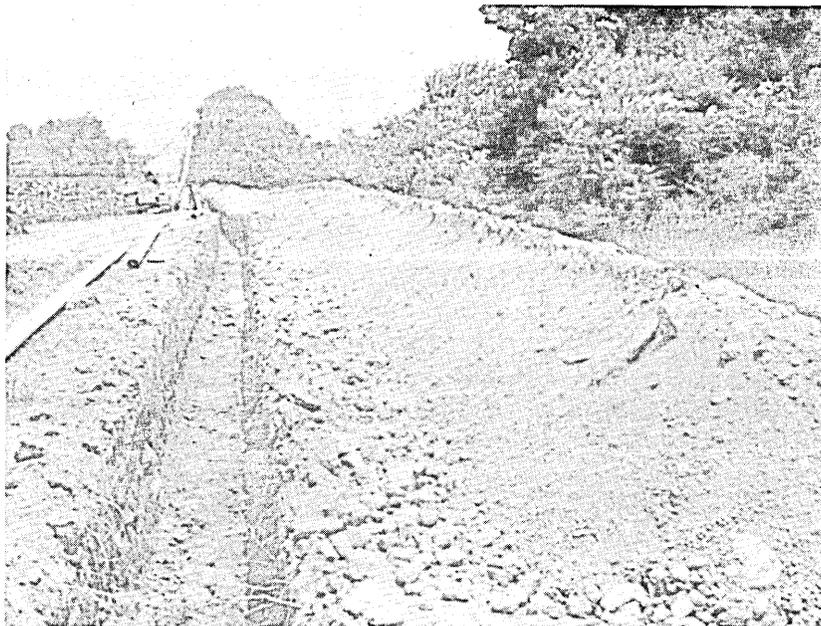
Fig. 7—Sheath strung along right of way.
