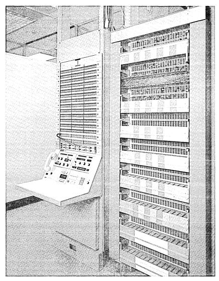
Fig. 5-950A testboard and cross-connect bay.
