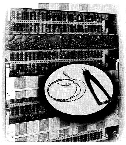
Fig. 7-Cross-connect panel, jumper, and removal tool.
