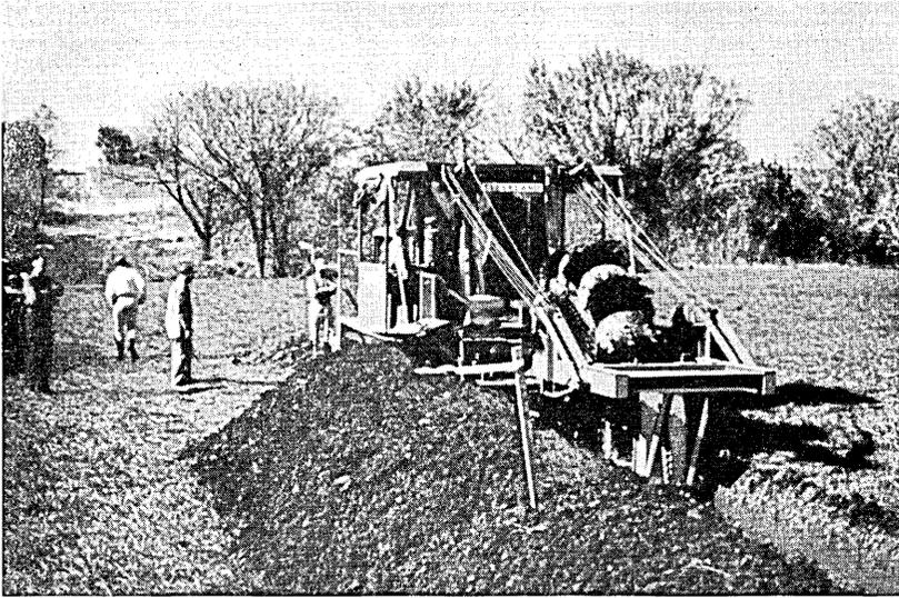
Fig. 6 — Trenching: four foot depth.
