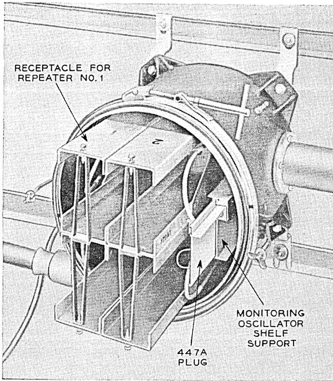
Fig. 17 — Basic repeater apparatus case with cover removed, mounted on the manhole wall.
