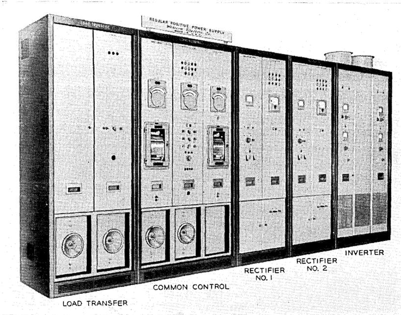
Fig. 3 — Terminal plant — regular power supply.
