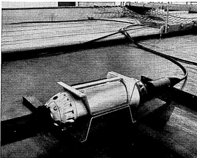
Fig. 4 — Repeater clamped in individual rack framework.
