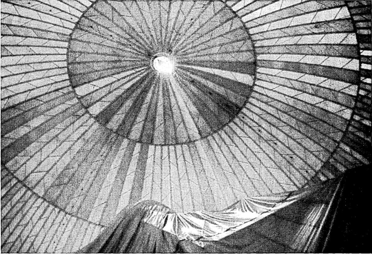
Fig. 26 — Upward view showing herringbone pattern inside Andover radome.
