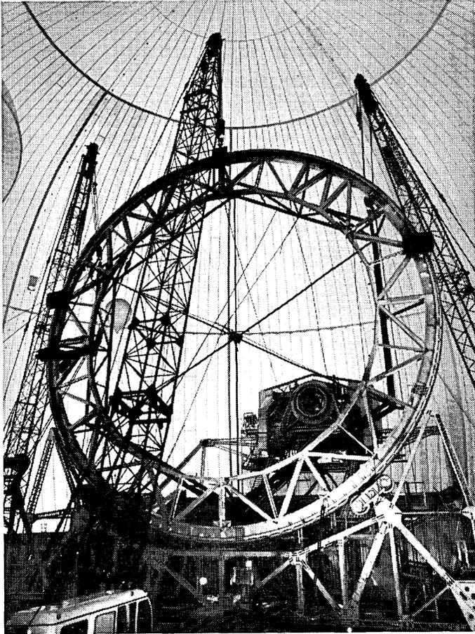
Fig. 9 — Final phase of installation of elevation wheel.
