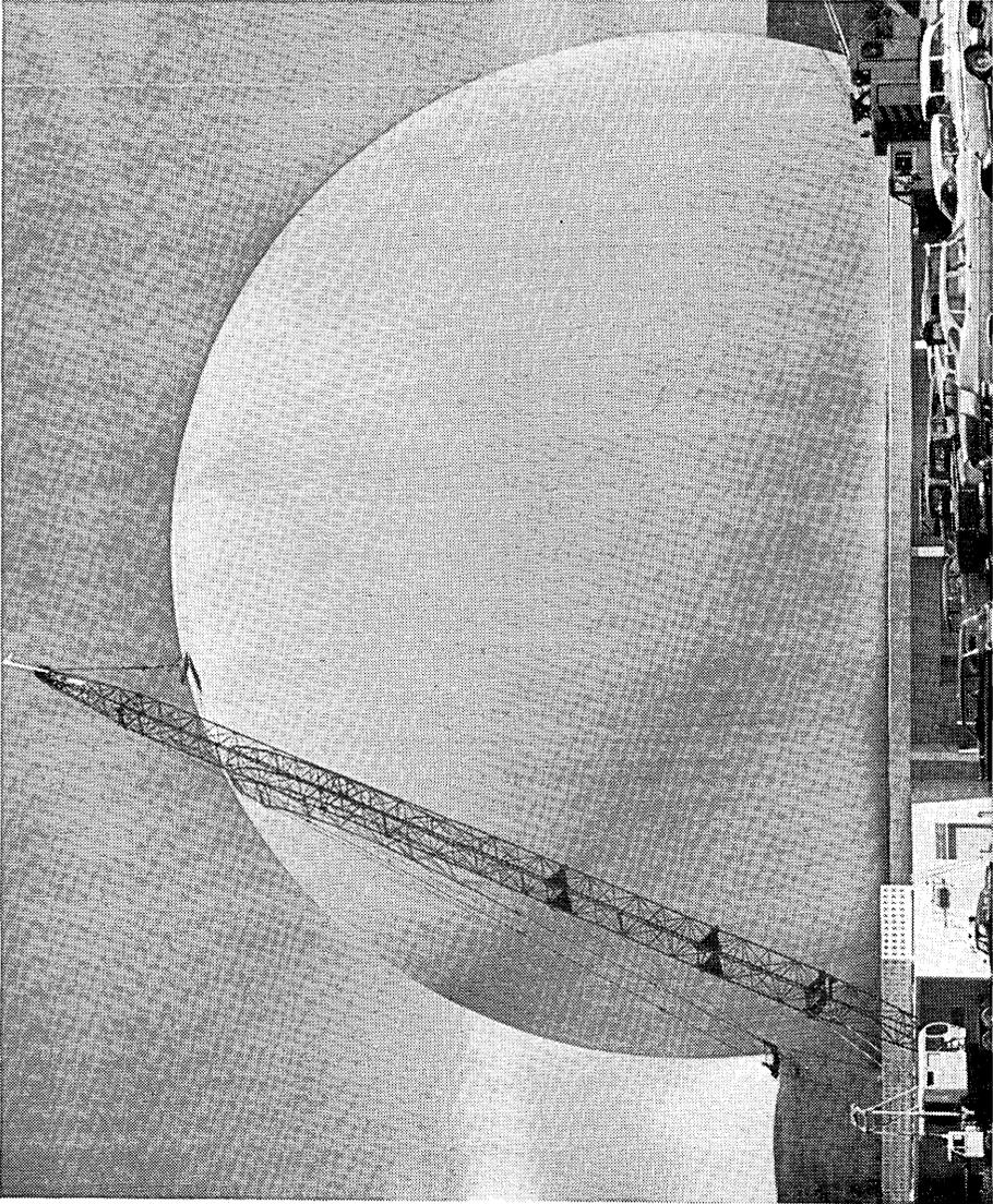
Fig. 31 — Radome installation complete and fully inflated.
