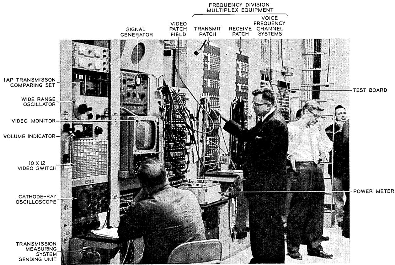
Fig. 5 — Portion of Andover test area.
