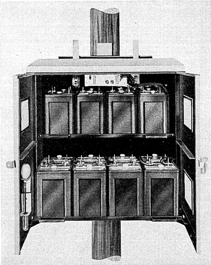
Fig. 25 — Primary battery power plant.
