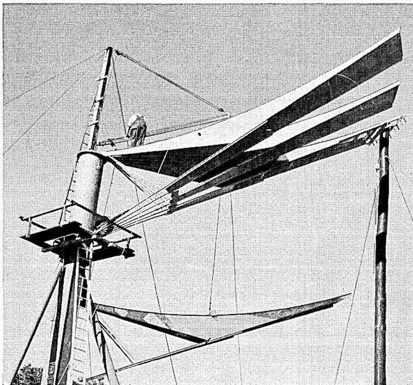
Fig. 1 — Fastening the radial sectors to the hub.
