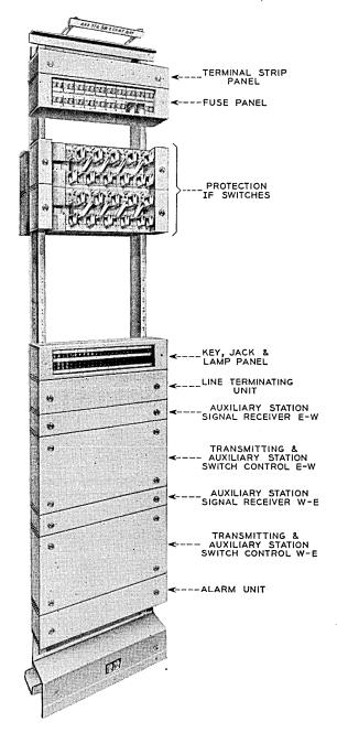
Fig. 16 — Auxiliary station switching and control bay.
