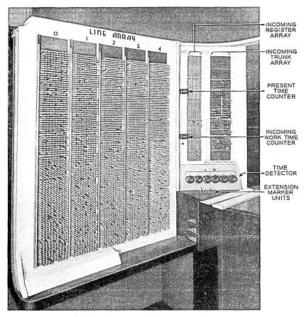
Fig. 16-Originating position-left side.
