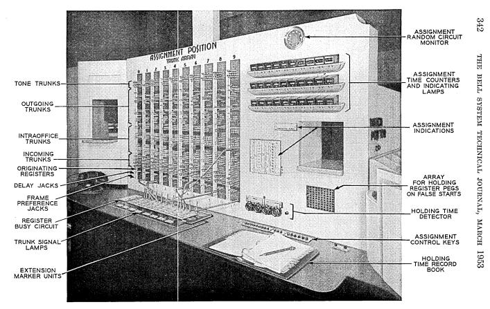
Fig. 21-Assignment position.
